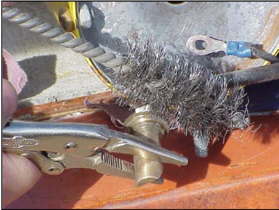
Figure 4. Corrosion on electrode. Use a wire brush, emery cloth or similar abrasive material to remove corrosion from point where electrode contacts the rear cover.
